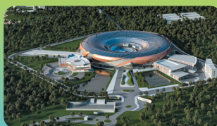
SPS-II, Rayong, Thailand 3 GeV
