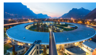
ESRF-U, Grenoble, France
